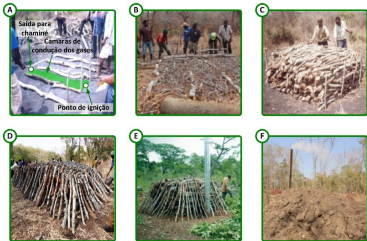
Figure 4: Construction stages of the IBEK kiln (Martins, 2016) 24
